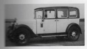
E 1930-32 (prod: 10,943). 2-seater, coupé, fabric saloon, various F.R. 1861cc (S4 SV). Indestructible old fathead (born 1921) giving 27bhp at magneto ignition, transmission and artillery wheels, but now with magnetor shell, chromium plate and ball change tour-speed 'box. Saloons re-styled for '31, no codies in '32 range, which latter will probably wheels, though artilleries still available.
