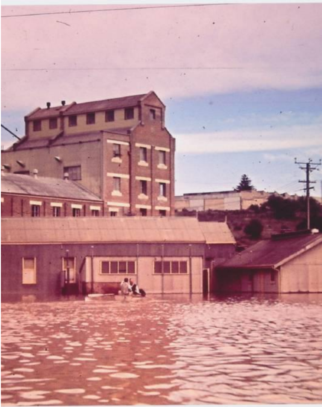
Murray Bridge in flood 1956
