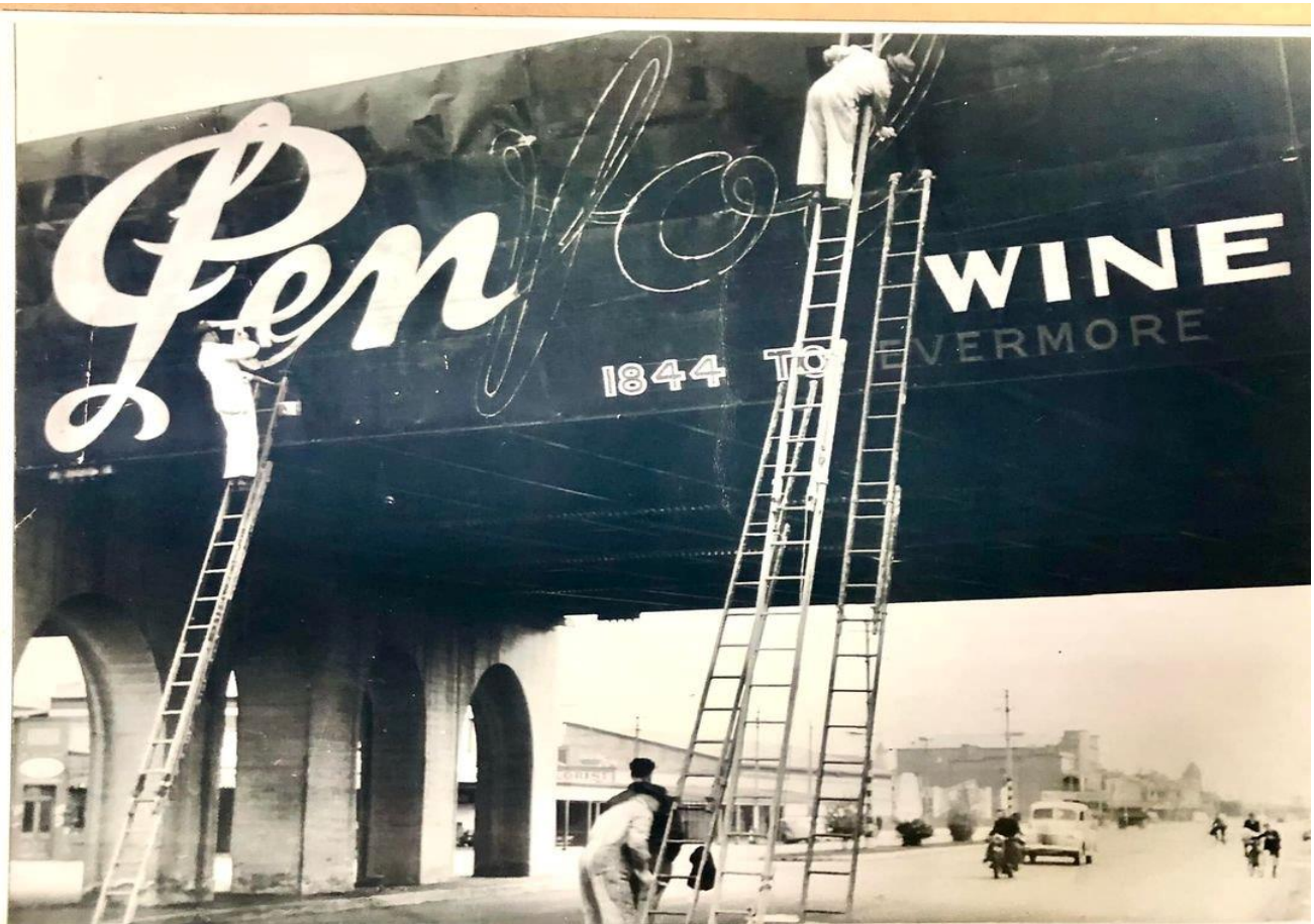
Port Adelaide Railway Bridge
